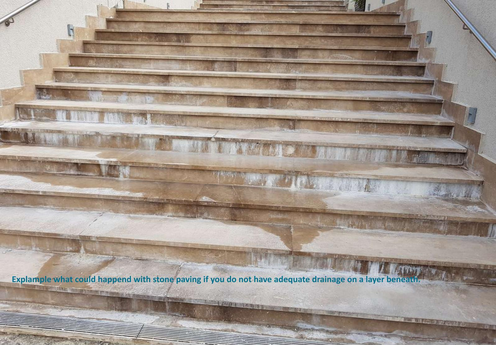
Example what could happen with stone paving if you do not have adequate drainage on a layer beneath.
